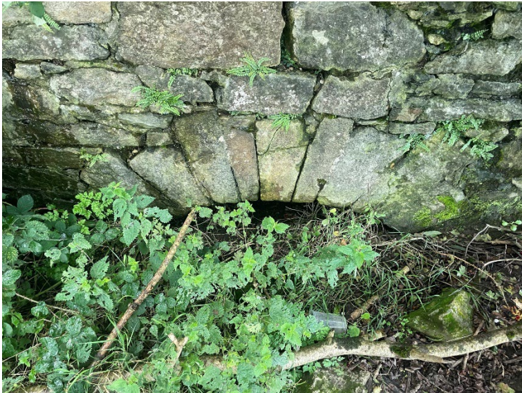
Figure 23 Flood relief arch to the North of the bridge
