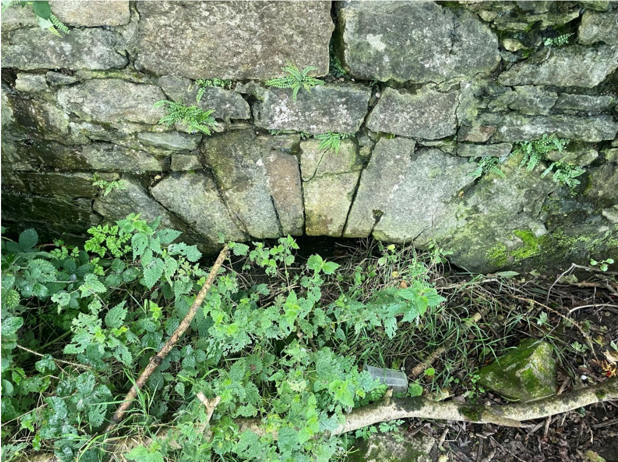
Figure 6: Flood relief arch to the North of the bridge
