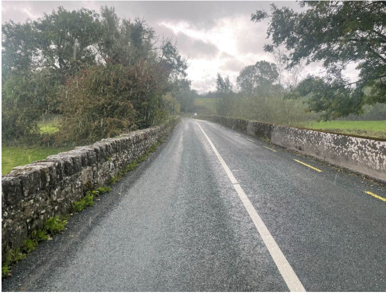
Figure 10 View to South along modern bridge surface.
