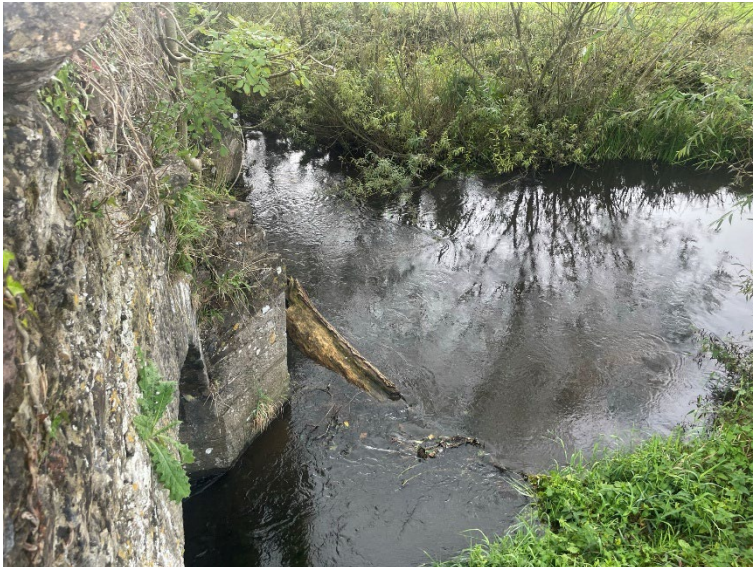
Figure 17 Upstream Ashlar Cutwater (CW-01).
