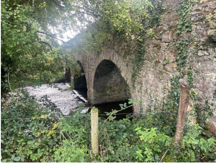
Figure 25 Downstream Arche elevation.
