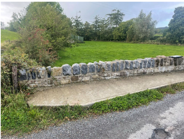
Figure 12 Section of modern masonry wall and concrete footpath.
