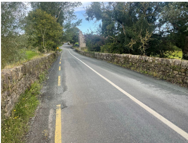
Figure 9 View to North along modern bridge surface.
