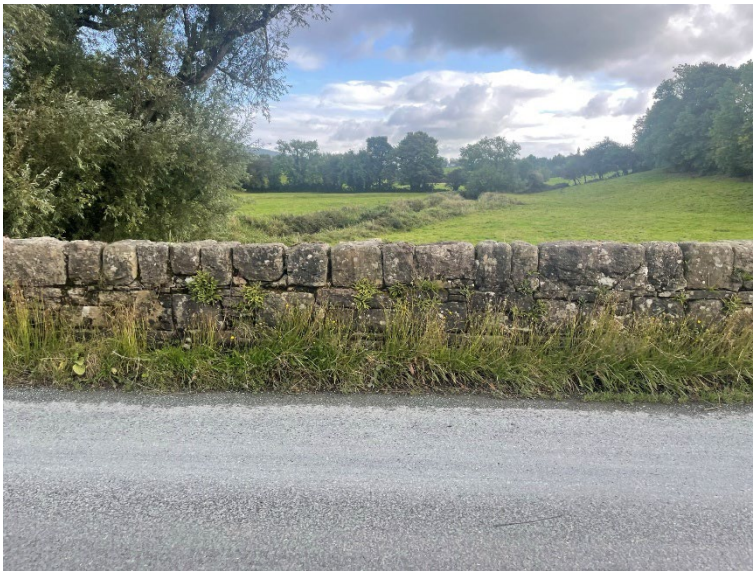
Figure 11 Internal face of Masonry Parapet
