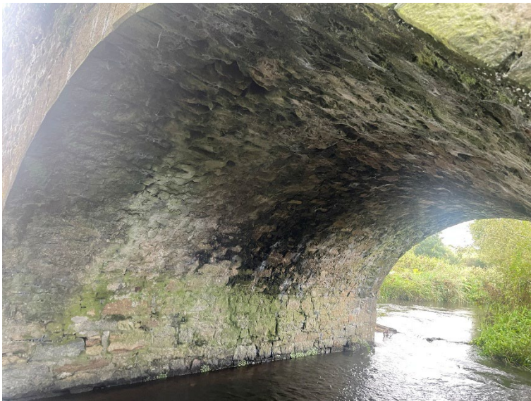
Figure 26 Underside of Arch 1 viewed from Downstream embankment.
