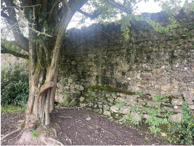
Figure 22 Downstream Bridge Wing Wall.
