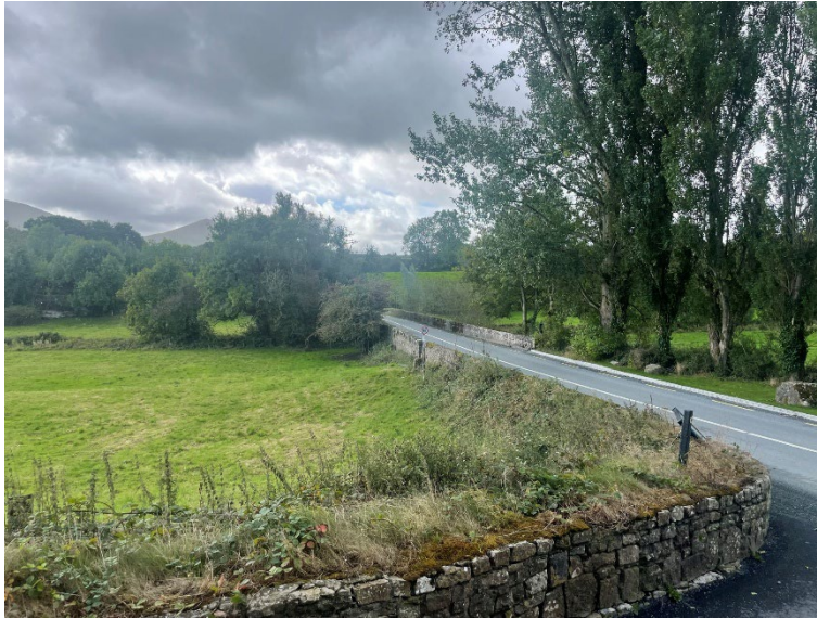
Figure 7 Galbally Bridge View from the North.
