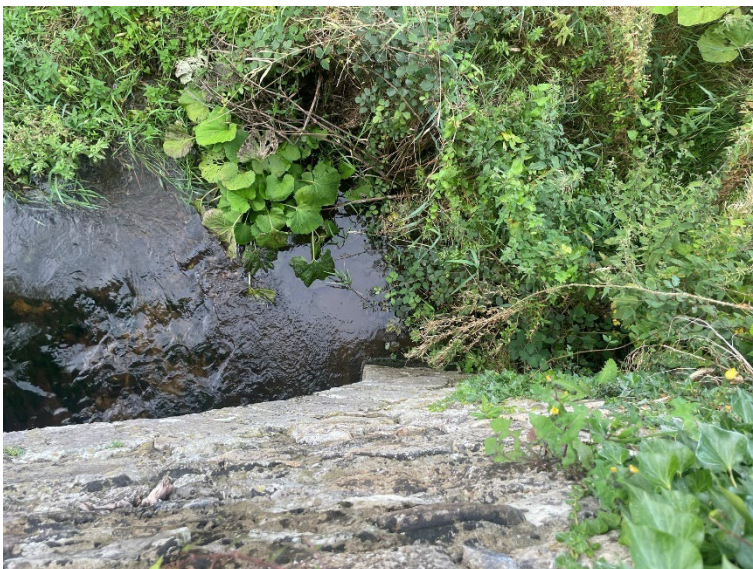
Figure 18 Upstream Bridge Abutment with vegetation growth.
