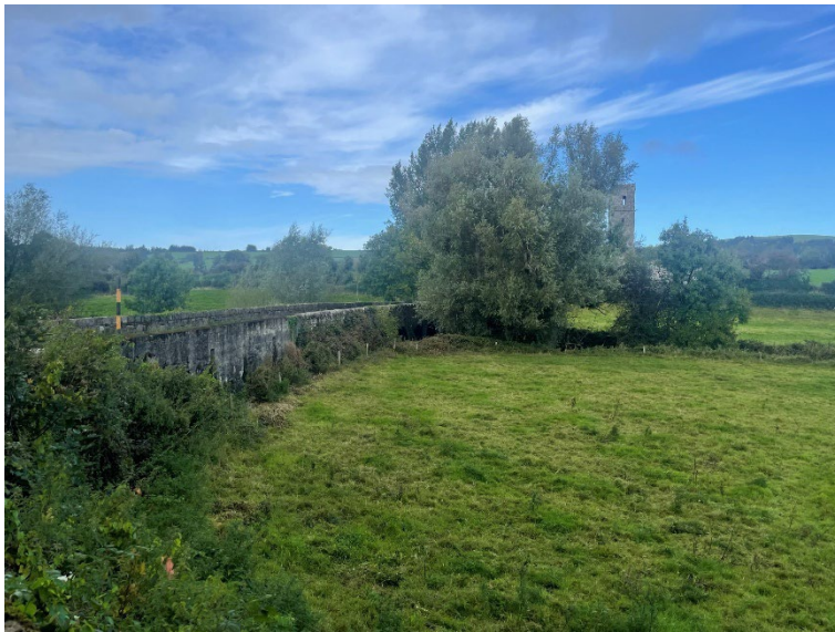
Figure 8 Galbally Bridge View from the South
